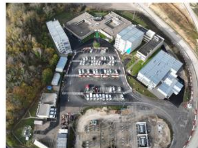
Installations de bases vies et restaurant inter-entreprises
