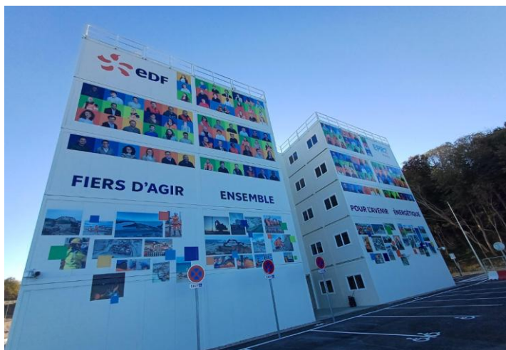
Installation de bases vies
