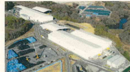
Soil reception / separation facility of Interim Storage Facility (Okuma Town)
