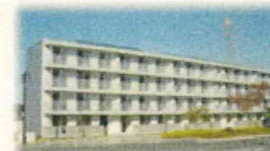
Hiwada housing complex, reconstruction public housing managed by the prefecture
